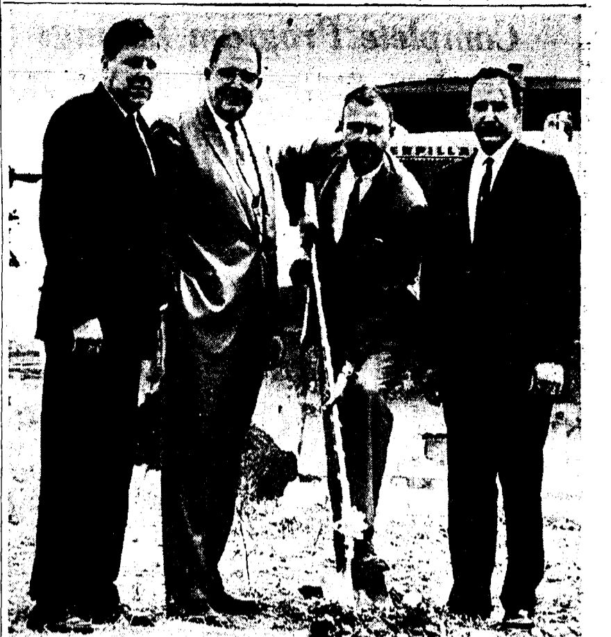
VIKING BREAKS GROUND — The start of Viking's $750,000, 126,480 sq. ft. cable manufacturing plant in Freehold Township is marked as Theodore Baum, Viking executive vice president and treasurer, applies the shovel. From left, Donald F. Wood, Freehold Township Planning Board chairman; Myron Taylor, Monmouth County Planning Board Industrial Representative, and, far right, Howard Ruveda, Viking plant manager.
