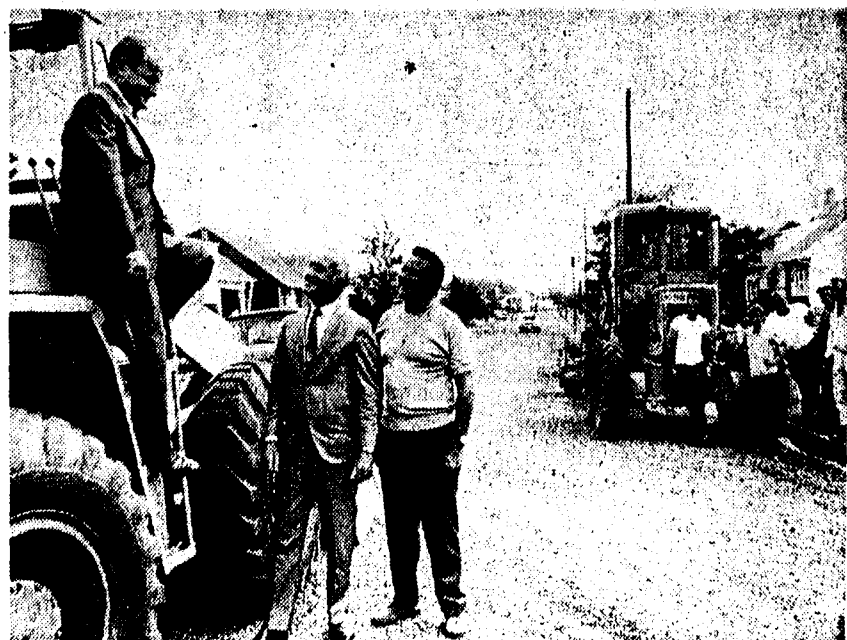
ACCOMPLISHED MILESTONE —Union Beach Mayor Alfred T. Hennessy Jr. steps down from front-end loader being used in construction of hard surfaced roads throughout the borough. Construction is going so well that Councilman Arthur Lembo, right foreground, will ask council for additional funds to speed up the project, designated as a five-year plan. Borough Engineer Edward Reilly, center, also turned out to inspect work on Scholer Drive. Borough employees in background take advantage of the brief respite. (Register Staff Photo)
