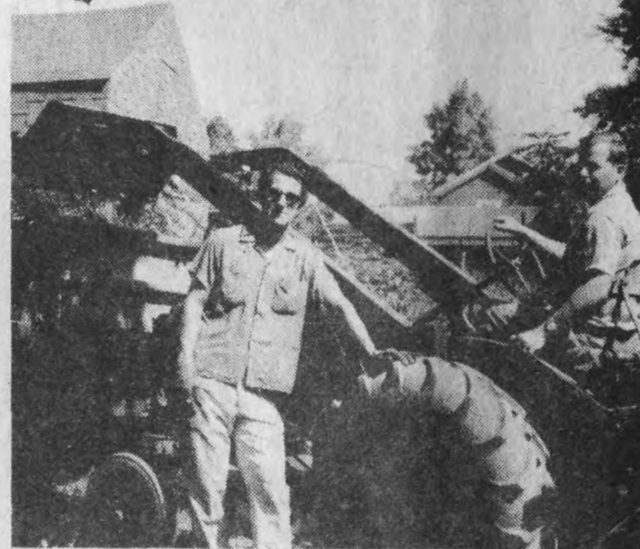
Ray Skotek, left, and Daniel Martin Load debris into Truck.
