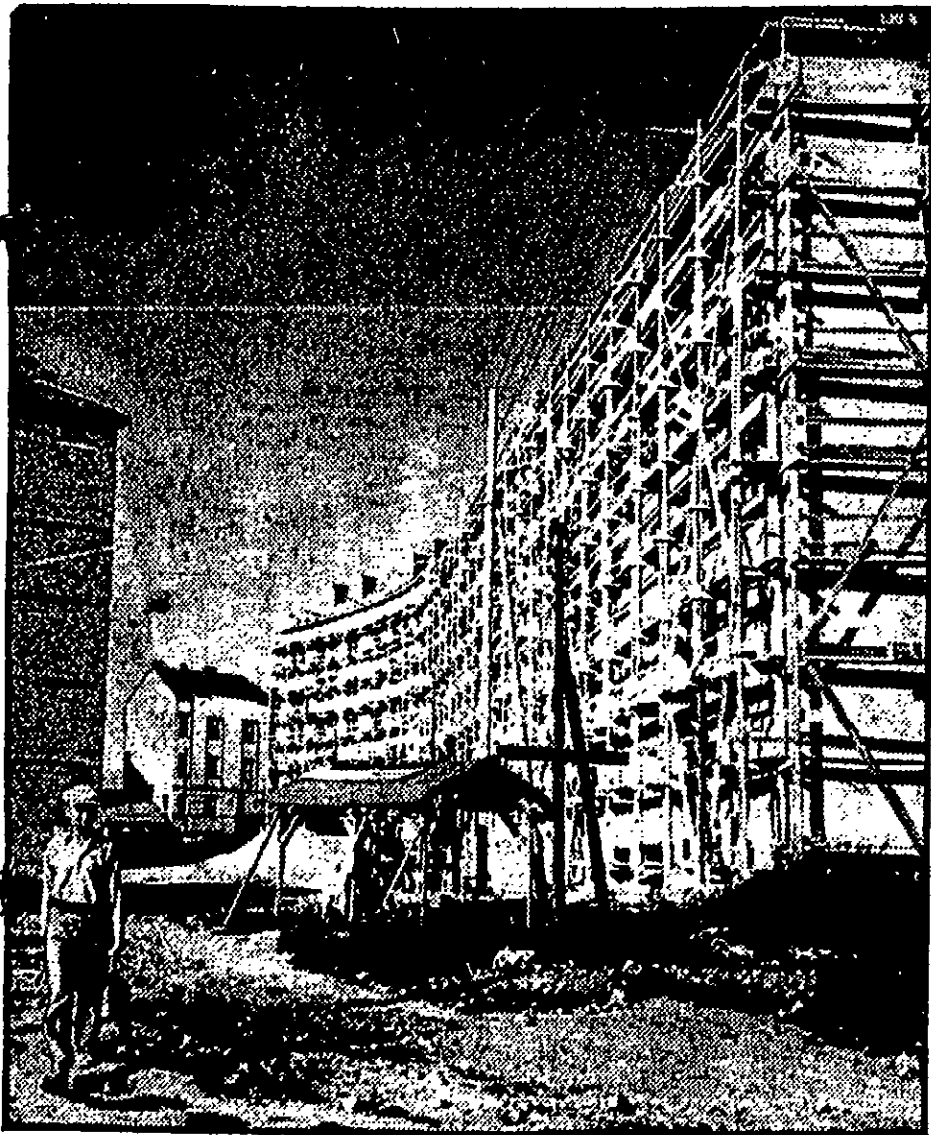
The accent in the land of Tito these days is on work. Yugoslav men, women and children share the arduous task of rebuilding and modernizing their war-torn homeland. These new workers' flats are being built to replace bombed-out apartments in Belgrade. They contain two and three rooms and will house from four to six persons.
