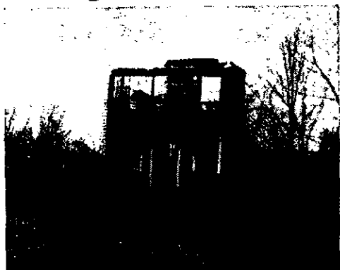
CHARRED SKELETON—All that remains of the Mack home on Easton Ave., where four youngsters lost their lives last Friday morning, is this blackened outline of what once was a home.
