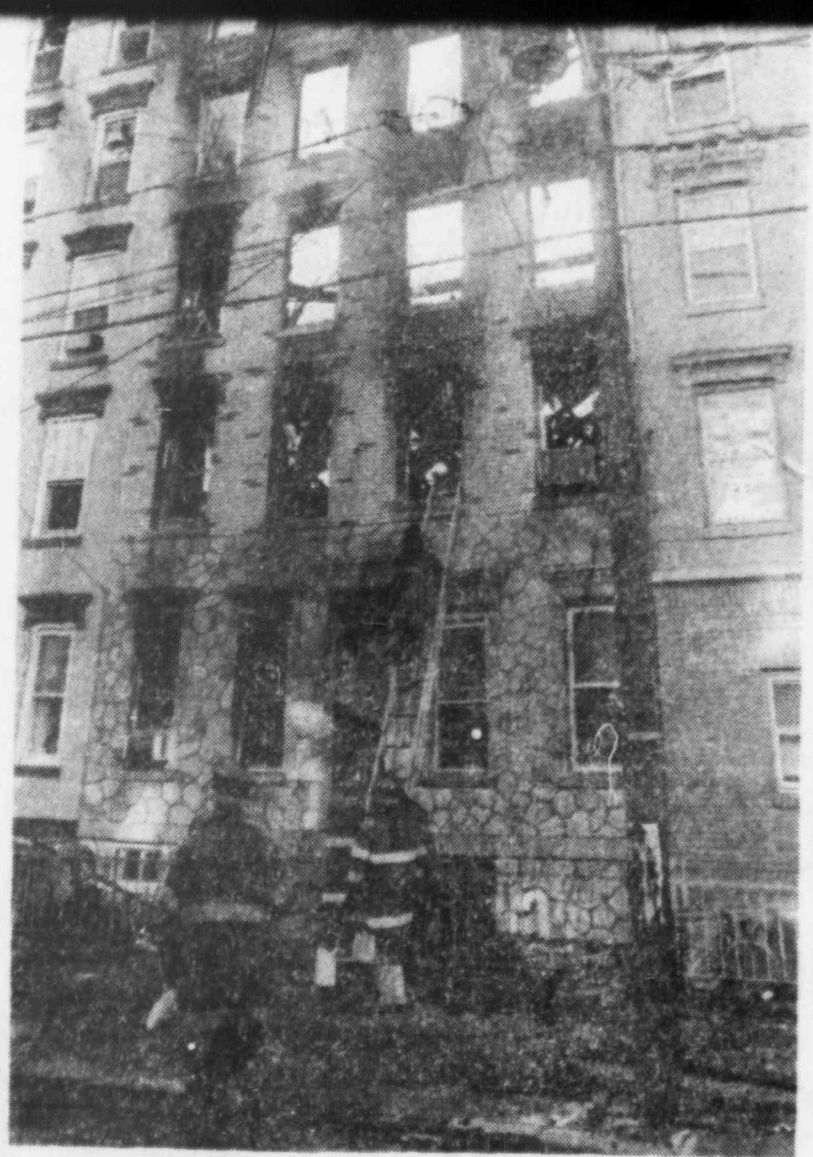
Hoboken firefighters inspect the ruins yesterday afternoon of early-morning blaze at 121 Willow Ave. DON SMITH/THE HUDSON DISPATCH
