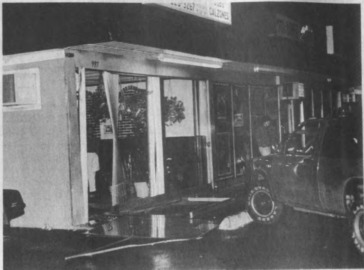
Nina's Pizzeria at 997 Amboy Avenue became an instant drive-in restaurant the night of February 11 when this 1987 pickup truck entered the premises through the front plate glass window. Witnesses said the driver backed out of the building as fast as she drove into it. Wendy A. Koseski, 18, of 1035 Amboy Avenue, told Edison Patrolman David Orosz she was pulling into a space in front of the restaurant when her foot slipped off the brake and onto the gas pedal. This, reported Orosz, propelled the truck into the building, smashing the entire front. Koseski was charged with careless driving.
