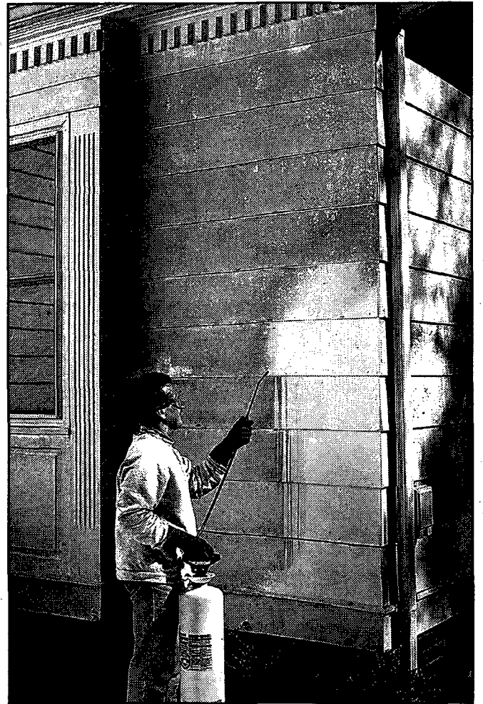
Kill mold and mildew on contact with Jomax, which contains an EPA-registered mildewcide.
