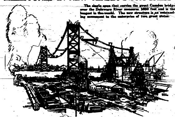
THE great cables that will support the sixty-foot roadway over the Delaware are being rapidly laid and the completion of this highway between New Jersey and Pennsylvania is now a matter of months. Current furnished by Public Service Electric
