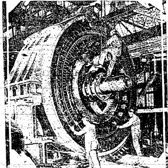
Eight big motors, each rated at 22,500 horse power, will propel the powerful and speedy alruhane carrier Lexington now under construction at Quincy Mass. The motors are 15 feet in diameter and weigh 222,000 pounds each.
