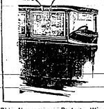
Old Newspapers Protect Window Glass While Painting a Car. drivers to be careful is one of the most | edges of the glass, leaving none of it important features of the accident exposed. When the fenders are to be
