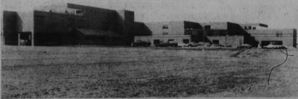
NEW MIDDLE SCHOOL — This is the new $7.4 million middle school in Marlboro which will be dedicated tomorrow. The school, which has been in
