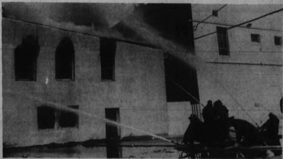
TOTAL LOSS — Police and fire officials, who yesterday ventured into the still-smoking ruins of the Morris Building, rear portion of which shown above, at 715 Mattison Ave., Asbury Park, say the Wednesday fire left the structure beyond repair.
