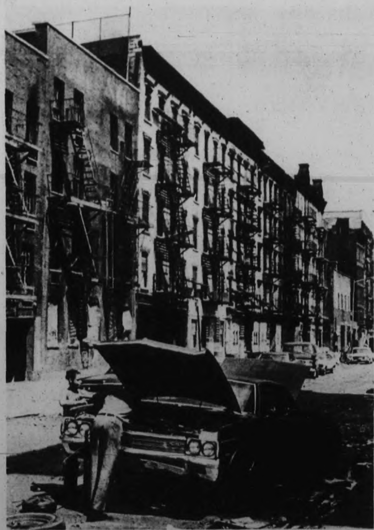
URBAN PROBLEM — A New York tenement block like this one may turn out to be the beachhead for review of federal urban policy.
