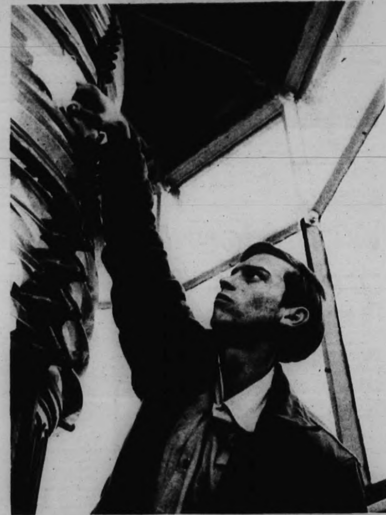
LIGHTING UP THE HOOK — Seaman Richard Guy of Station Sandy Hook cleans the lens of Sandy Hook Light. The light in this tower was first used on June 11, 1764. Today, it uses a 60,000 candlepower electric light mounted in a white stone tower 88-feet above the water. It is visible for 15 miles.
