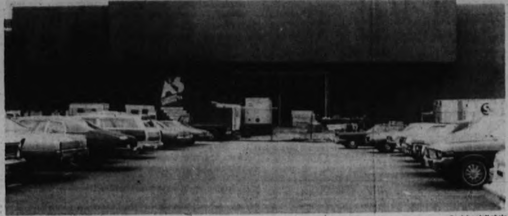
COUNTDOWN — Signs at construction site of new Abraham and Straus store in the Monmouth Mall announce spring opening, a schedule A&S officials expect to meet with beefed-up construction crews and extra shifts.
