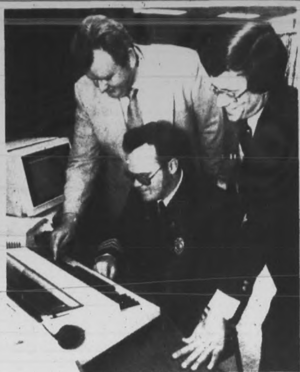
COMPUTER DONATION — Ed Smith, left, director of customer service at Syntrex Corp., oversees the installation of an AQUARIUS office automation workstation at Eatontown's Engine and Truck and Hose Company 1, while First Assistant Chief Alan Trask, center, sits at the terminal, and Fire Commissioner Theodore Lewis, who also is council president, watches.
