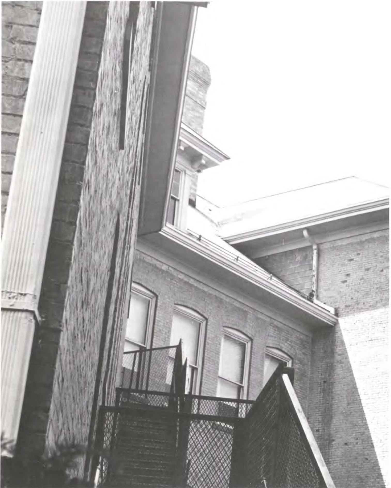
Branch Avenue Building
