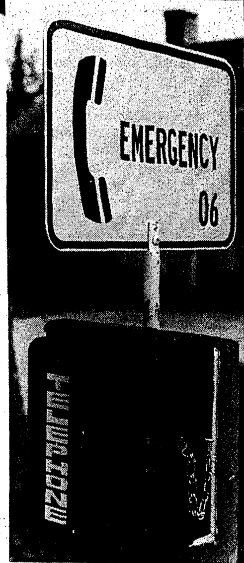
New call boxes, like this one in front of the Community House, are topped by numbered signs. (Above) Police dispatcher Susan Holtz answers a test call from an emergency phone.
