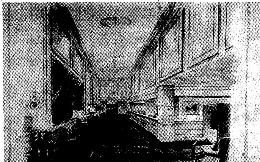
Entrance lobby to the Island Club at Sundial.
