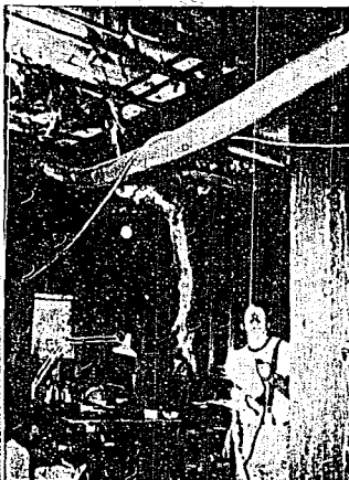
Sanibel fireman Don Frye inspects the damage from this week's fire at the residence of John Eichenlaub — the second damaging fire on the island in a one-week period.
