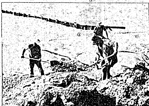
Dick Holmberg and his crew at work on the perpendicular stabilization project, which was completed this past weekend.
