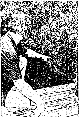
Dave Wooster points to some of the erosion problems along the canal behind his house on Dixie Beach Boulevard.
