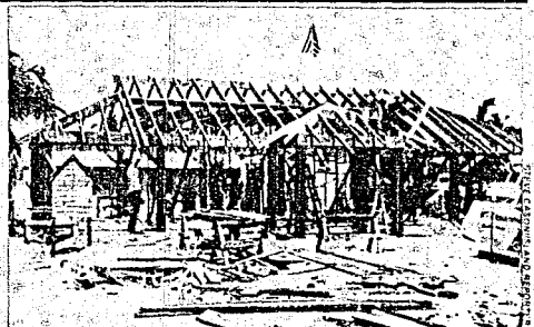
Construction crews work to complete Gramma Dol's snack bar at Sanibel Marina. The inn is supposed to be completed by Aug. 15, but marina owner Milton Ireland said work might not be finished until the end of the month.
