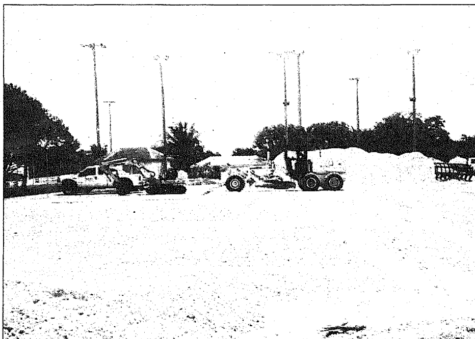
Construction crews removed the tennis courts at The Sanibel School
