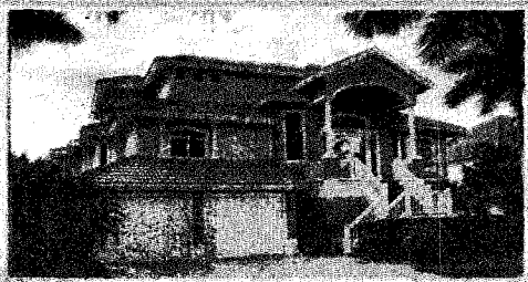
BEACHVIEW Lavishly renovated in 2008. This 4,657 sf under air, 2-story, 4/3.5 pool home has everything you could want, incl. golf and more! Better than new offered at $1,895,000
