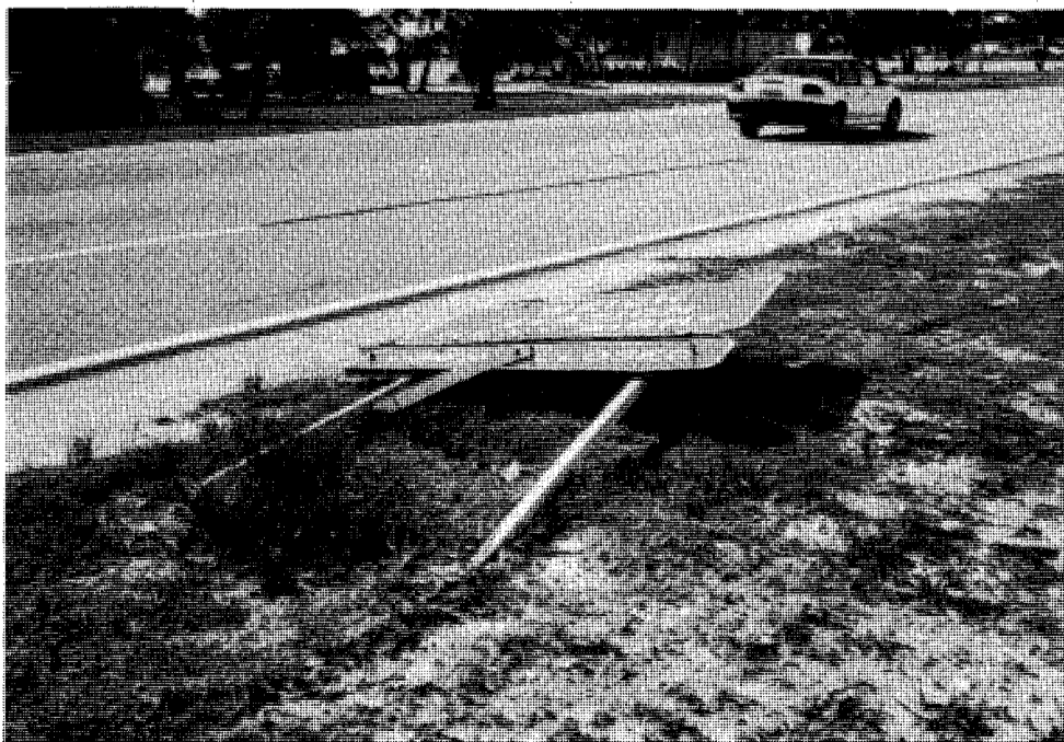
Gusting winds from Hurricane Andrew knocked down the weigh station sign on the causeway.
