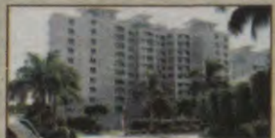
FORT MYERS BEACH Starting at $380,000 Waterside Condominiums
