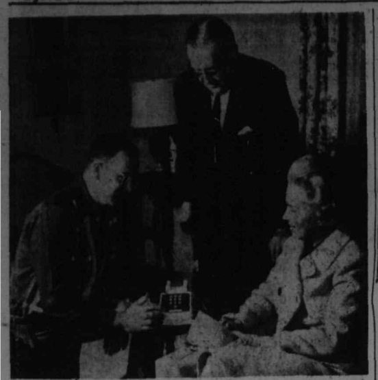
FIRST WITH THE LATEST —Ray Kerrigan, New Jersey Bell Telephone Co., left, installs touch-tone telephone at the home of Mr. and Mrs. Harold T. Graves, jr., 29 Whitredge road. Touch-tone service, which features push-button instead of dial telephones, made its New Jersey debut in the Summit-Chatham area this week. Graves is president of Summit Trust Co.
