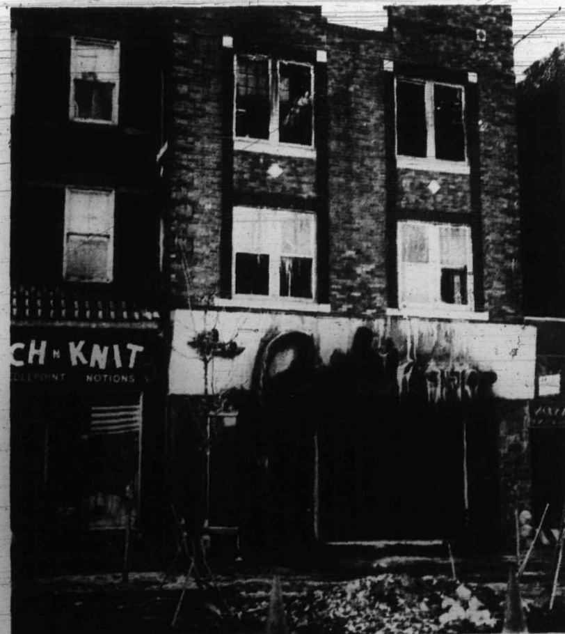
DAY AFTER THE NIGHT BEFORE - The Kern Building at 422 Springfield avenue, including the Babs Shop, lay in ruins Tuesday morning in the aftermath of Monday night's fire that completely gutted the structure. The fire raged for nearly three hours before it was brought under control shortly after 11 p.m. (Wolfin Photo)
