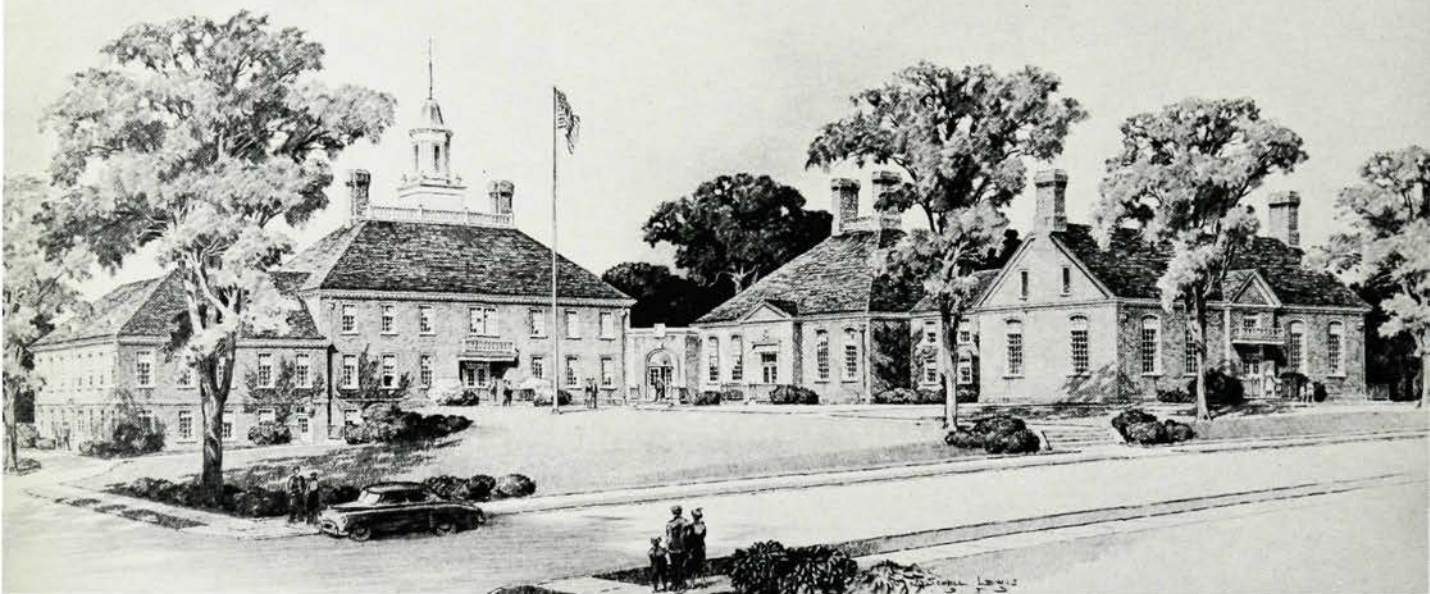
On an attractive plot directly off Mindowaskin Park, the Municipal Hall is of old Williamsburg style.
