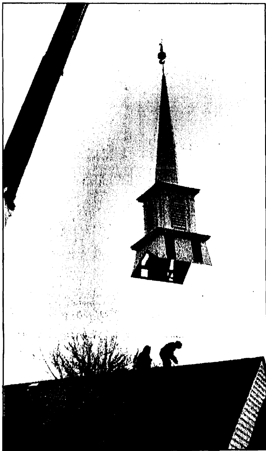
The new steeple is lowered into place at Willow Grove Presbyterian Church in Scotch Plains.
