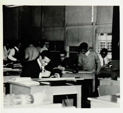
Templates, compasses, and T-squares are used on the drafting boards in the making of blueprints, perspectives, and machine drawings.
