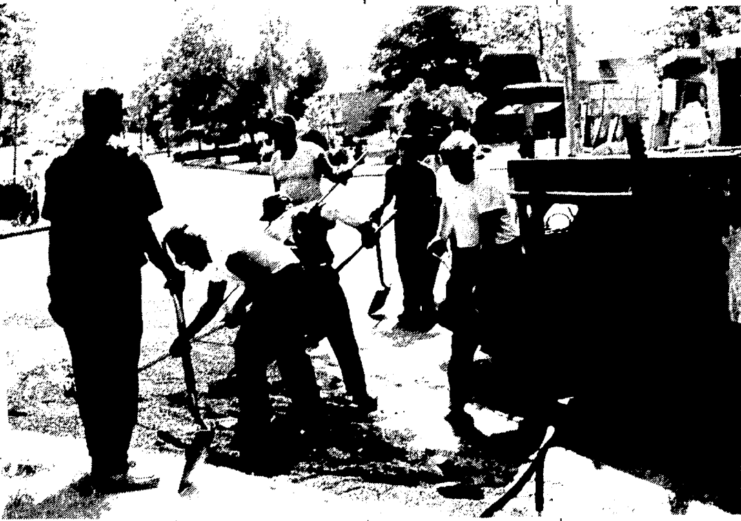
Walter Hamlette's road crew has been hard at work on the annual August paving program. Traditionally scheduled during vacation period when disruption is minimal, the paving process also requires August's hot weather in order for the tar to "cure" properly. Supervisor of Maintenance and Construction Dan Kelly noted, "Although our post-storm cleanup has been delayed, any postponement of the paving could interfere with residents returning to full work schedules and children going back to school."
