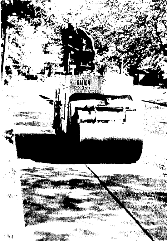
Walter Hamlette's road crew has been hard at work on the annual August paving program. Traditionally scheduled during vacation period when disruption is minimal, the paving process also requires August's hot weather in order for the tar to "cure" properly. Supervisor of Maintenance and Construction Dan Kelly noted, "Although our post-storm cleanup has been delayed, any postponement of the paving could interfere with residents returning to full work schedules and children going back to school."
