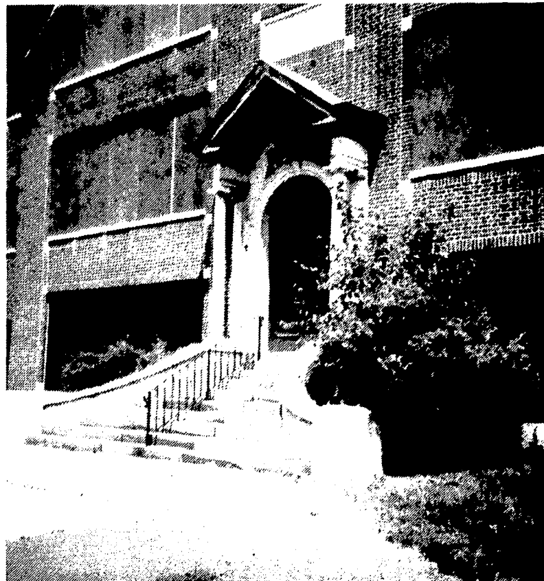
The former Holy Trinity Elementary School building on Trinity Pl., vacant for two years, will soon be on the auction block. The New Jersey Commission for Blind, which purchased the property, no longer intends to use it for its program for visually impaired.
