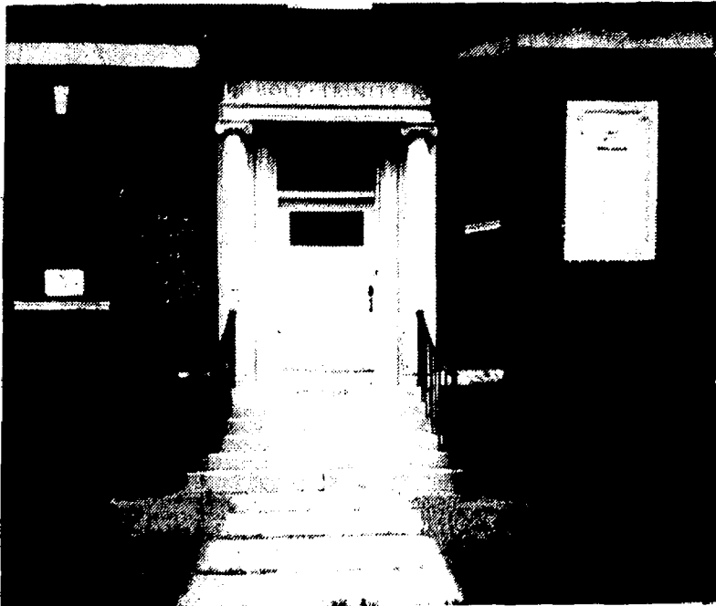
Holy Trinity's former parish convent, located on Trinity Pl., is one of three buildings now owned by the State. It too is boarded up as the result of vandalism.
