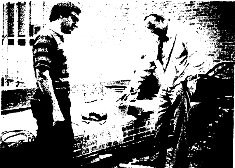
Clerk of the Works Jack Courter points to work being done to reroof the annex at Roosevelt Junior High School as school board member, Bill Vincentsen, chairman of the operations and facilities committee, looks on. Courter is employed by the school board to oversee roofing work being done at the junior high school.
