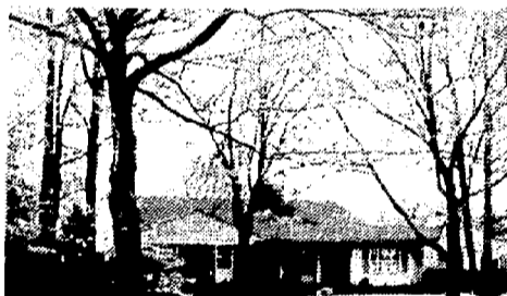
Weichert Realtors, 185 Elm St., Westfield, has announced the sale of the above property at 727 Tuxford Turn, Westfield. The home was marketed by Carol Lyons.
