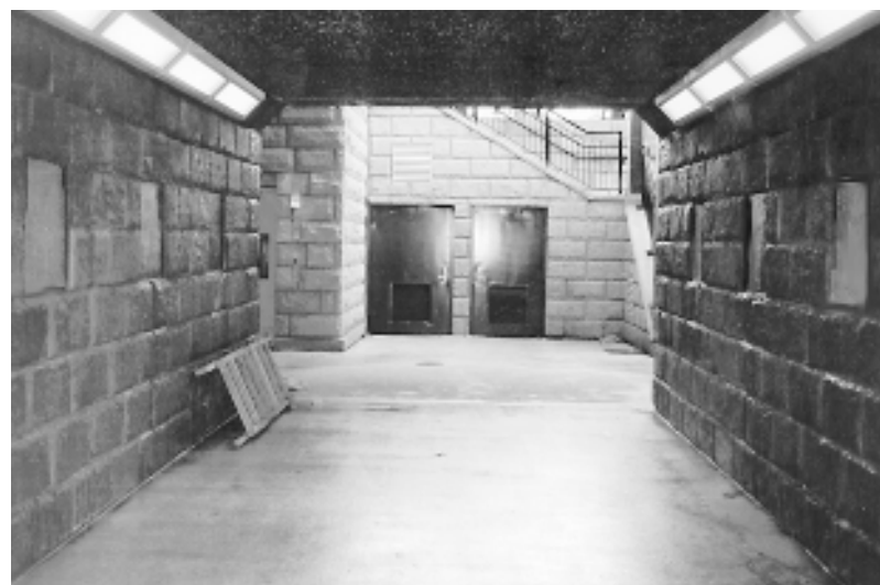
David B. Corbin for The Westfield Leader READY FOR COMMUTERS... The new pedestrian tunnel at the Westfield railroad station will be open to town residents this week. The tunnel is on the far left side of the station. The old tunnel will be permanently shut down.
