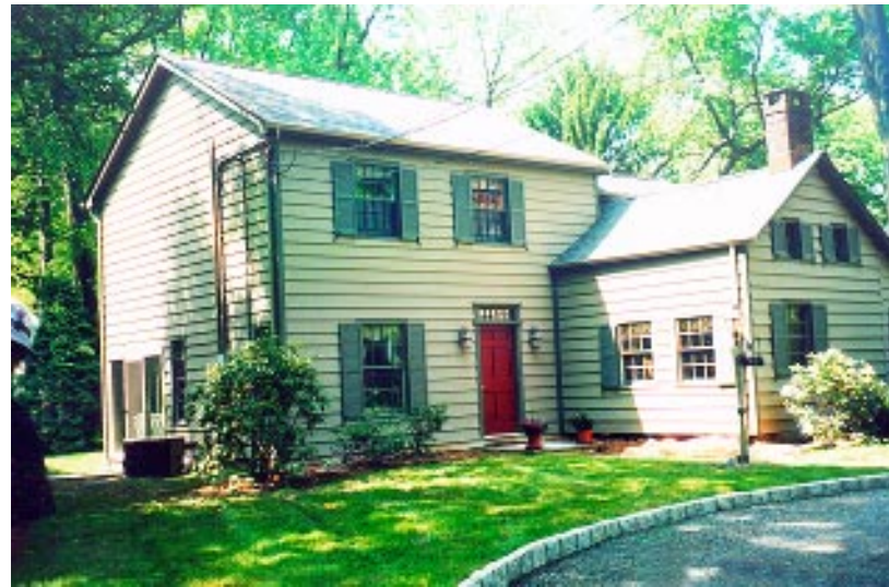
AN ADMIRABLE HOME...Mr. and Mrs. Larry G. Myers of 415 Woodland Avenue in Westfield will receive an award for the period addition, restoration and painting of their home during the Westfield Historic Preservation Commission's Sixth Annual Commendation Awards Reception, which will be held on Thursday, June 11, at 8 p.m. in the Town Council Chambers and Rotunda of the Westfield Municipal Building.
