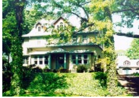
This home, at 521 Tremont Street and owned by Mr. and Mrs. John Walsh, was cited for extensive renovation.
