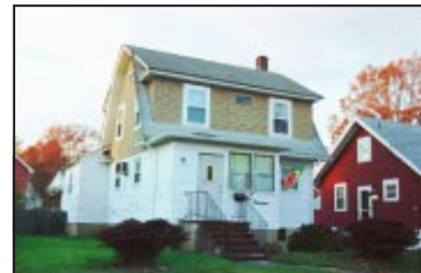
Coldwell Banker Schlott, Realtors, 209 Central Avenue, Westfield has announced its participation in the sale of the above property at 114 Benjamin Street, Cranford. The property was handled by Bob Devlin.
