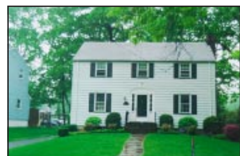
Burgdorff Realtors ERA, 600 North Avenue, West, Westfield, has announced the sale of 711 Willow Street, Cranford. The property was marketed by Faith Maricic.
