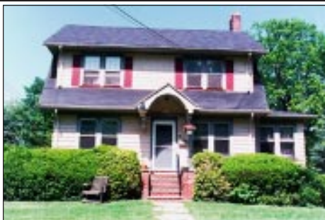
Coldwell Banker Schlott, Realtors, 209 Central Avenue, Westfield has announced the sale of the above property at 6 Sylvester Street, Cranford. The property was handled by Elvira Ardrey.
