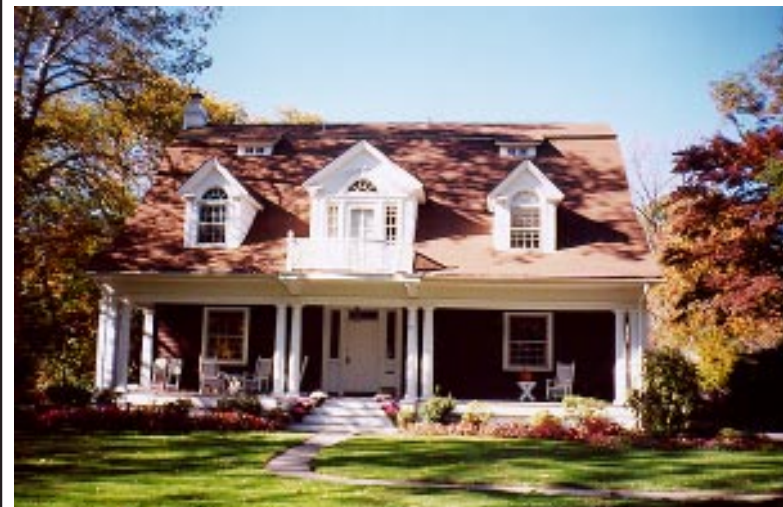
HOLIDAY HOUSE... This Stoneleigh Park home will be decorated by members of the Rake and Hoe Garden Club of Westfield as a "Cranberry Christmas" for the club's holiday house tour on Saturday, December 5. The turn-of-the-century architecture will be highlighted with natural plant materials, including grape vine trees accented with white pine, pine cones and cranberries. Tickets for the "Deck the Halls" tour of four Westfield homes and a holiday boutique are available from Rake and Hoe members and at Rorden Realty, Periwinkle's Fine Gifts, Lancaster, Ltd. and Clyne & Murphy.
