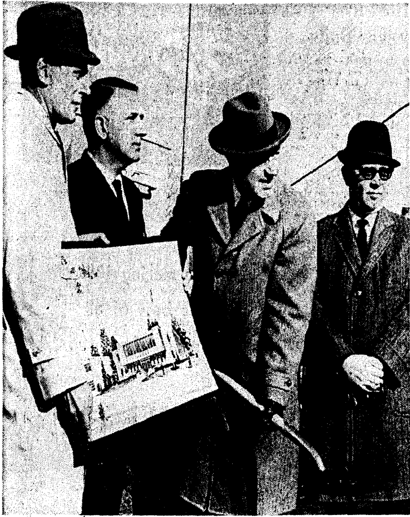
GROUNDBREAKING — Eatontown Councilmen Robert Dixon, left, and Bruce Mangan hold architect's rendering of the planned Eatontown municipal building. Mayor Herbert E. Werner wields a shovel in the groundbreaking at Broad and White Sts. Councilman Edward Clark is at right.
