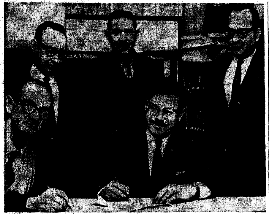
TEMPLE CONSTRUCTION UNDER WAY—Mortimer H. Zinn, right, seated, president of Congregation Bnai Shalom of Long Branch, and Graham E. Rockefeller of Rockefeller Construction Co. of Matawan, sign construction contracts for the congregation's new home on Lenox Ave. Onlookers are, left to right, Herbert Tanzman, Jacob Edelstein and Murray Weiss, all of the building committee.
