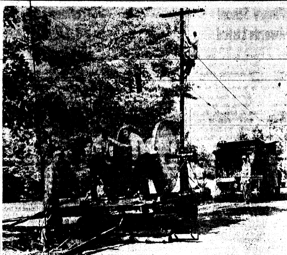
MORE POWER TO TOWNSHIP —Along Mountain Avenue this week Jersey Central Power & Light Co. crews are completing installation of new aerial cable feeding electric power into Blue Mountain area of New Providence Township. Last of mile-and-a-half, 5,000 volt, self-supporting cable is run off reel (above) preparatory to being pulled up and spliced. The new line, which will provide the Diamond Hill, Blue Mountain, Horseshoe and Ridge roads and Hillside Avenue sections with alternate power paths, is built of latest type overhead cable which, according to JCP&L, "operates very satisfactorily under the extremely bad tree conditions that prevail along these particular roadsides." Field work is under direction of Foreman Henry Long, Baltusrol road, veteran of 24 years' service with the utility in Summit.
