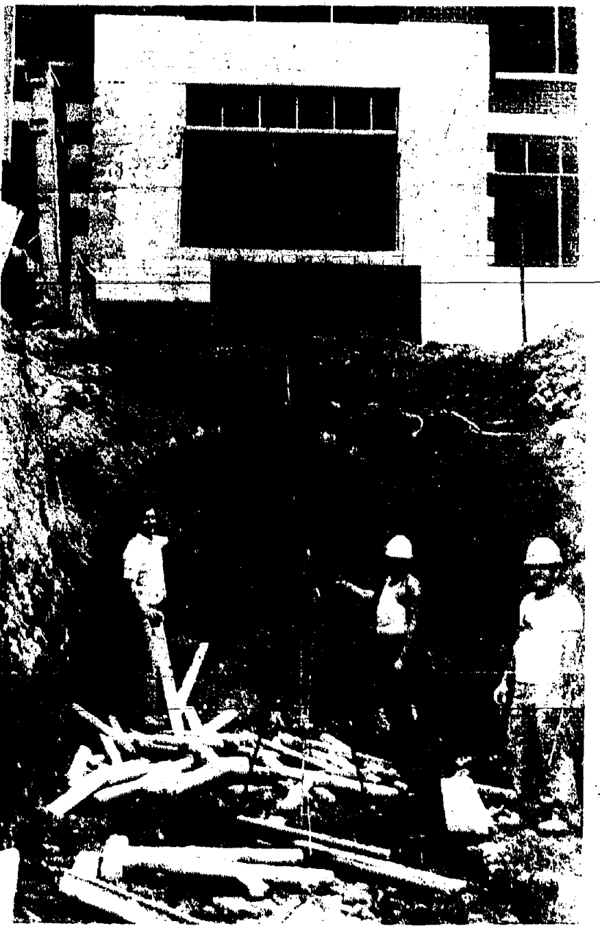
Old furnace cavity was unearthed in excavation for underground stormwater retention basin at Cleveland Plaza. It's from the old Alden Bigelow (Alden Street was named for him) mansion built on the site in the late 19th Century. Rick Rosencrantz of the Cranford Historical Society believes it was buried when mansion yielded to Cleveland School construction in 1913. Jose R. Carnadas of Spain, center, foreman for Seltzer construction, says it's well over 100 years old. He's flanked by Bernard Hughes, a Scott, at left, and Eladio Valdes, a Cuban, at right.
