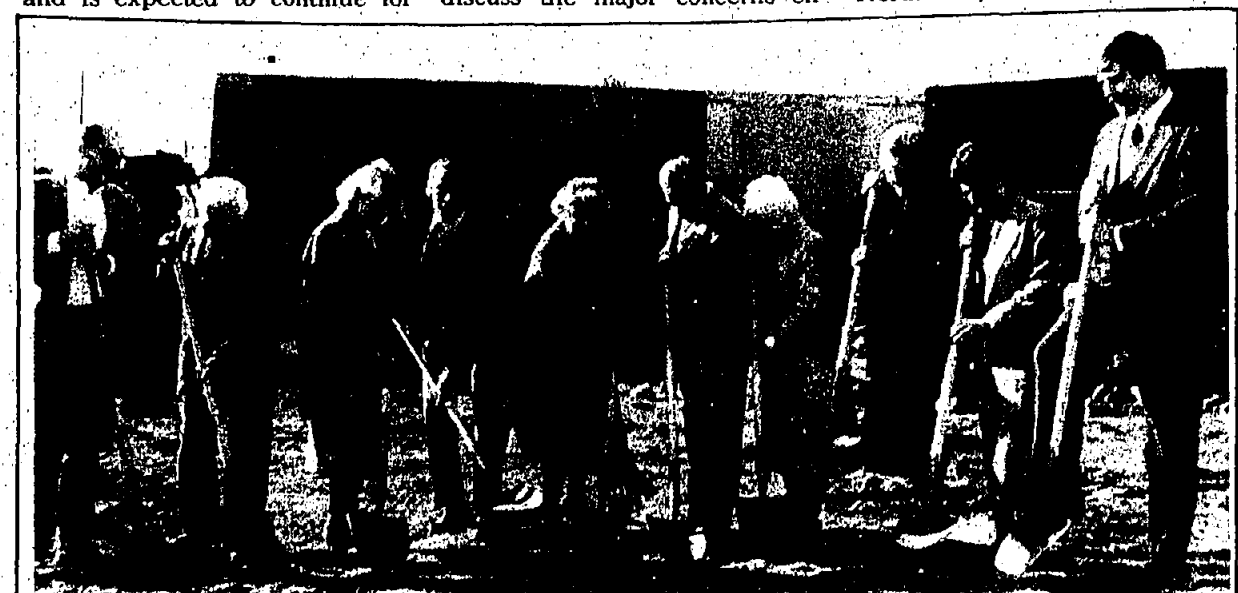
GROUND BREAKING: Breaking ground for new parking lot next to Cranford Library are, from left, Paul LaCorte, Vince Sarnowski, library director Penny Brome, Mayor Ed Force, Irma Miranta, trustees president Dan Swinton, Lois Swackhamer and Township Committee members Barbara Bilger, Carolyn Vollerio and Dan Aschenbach.
