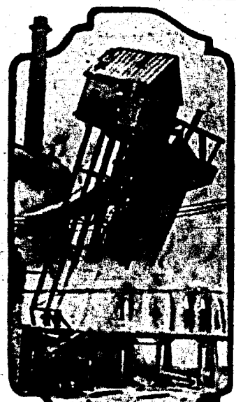
When the Pottstown, Pa., iron company decided to remove its old blast furnace and plant, constructed in 1880, to make room for new buildings, it thought that dismantling by sections was too slow. So 20 sticks of dynamite were used—and down to earth came the 500 tons of blast furnace.
