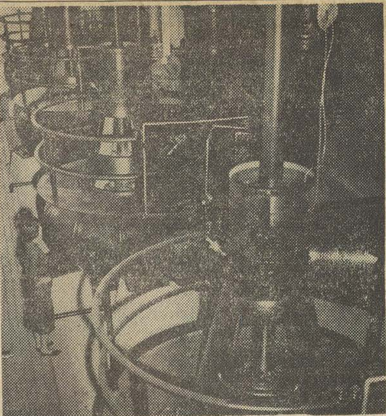
35 and 40 MGD pumps at river level.
