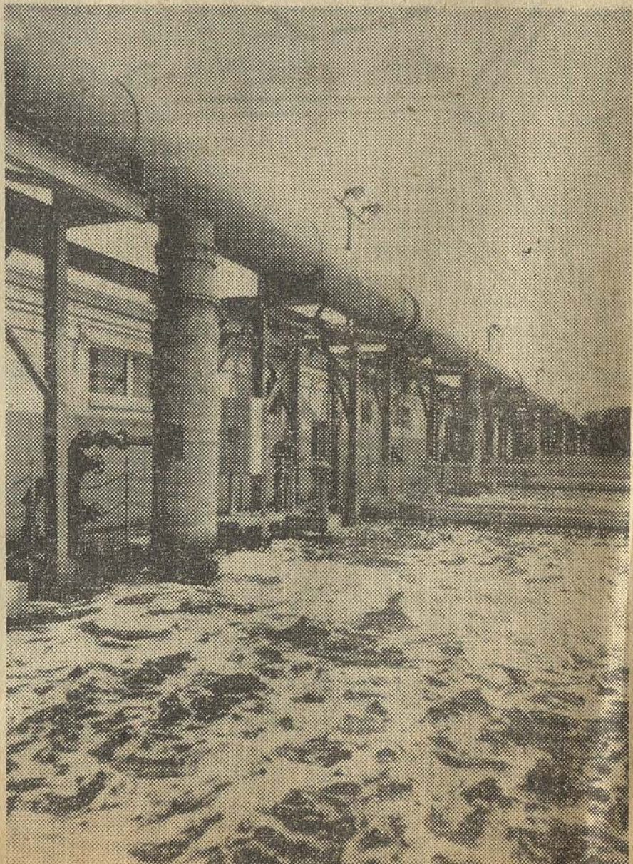
FULL SIZE—This shows a section of the six giant aeration tanks with overhead pipes which inject air into the waste mixture as part of the treatment at American Cyanamid. The watery mixture rolls to mix air and bacteria with the plant waste to eliminate pollution.
