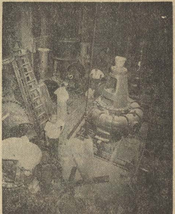
Suction and dispatch piping tie-ins to 40 MGD pumps.
