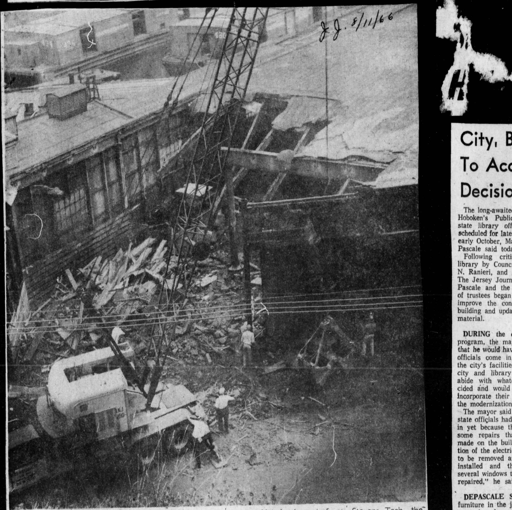
BIG BITE — Workmen move away the wreckage after a clamshell bucket has taken its bites out of the Long Dock on Hoboken's waterfront. Stevens Tech, the pier's new owners, will put up school buildings.
