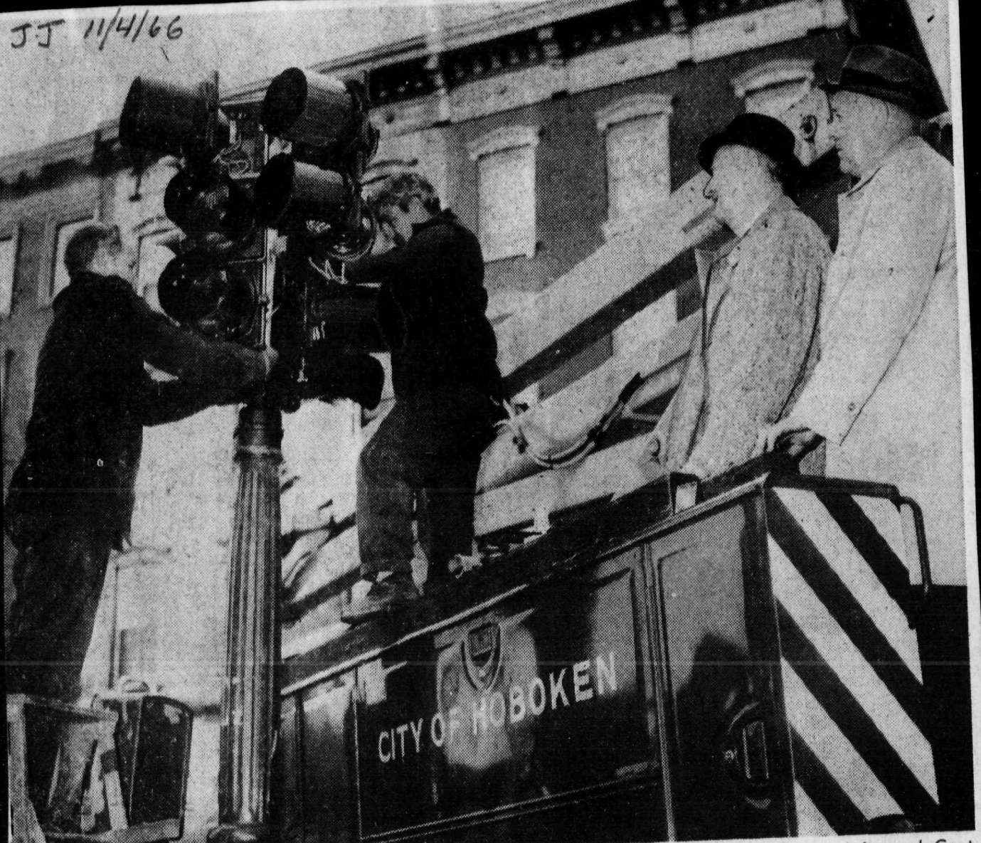
PARENTS URGE, CITY ACTS — Workmen install new four-way traffic light at 4th and Hudson Streets, Hoboken, after request by parents of children who use crossing daily. Work is being witnessed by E. Norman Wilson, public safety director, left, and Capt. George Baumann. Workmen from left are Arthur Wehrhahn and Michael Mazza. (Jersey Pictures)
