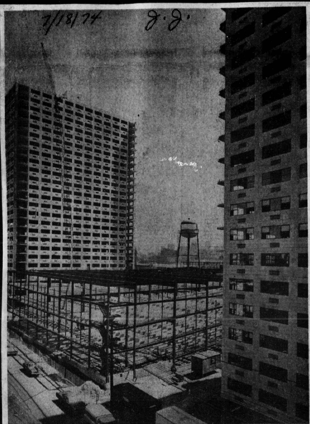
Steel framework for the first five-story parking garage at Grogan Plaza is completed. Twin 25-story apartment houses flanking the garage already have been enclosed.
