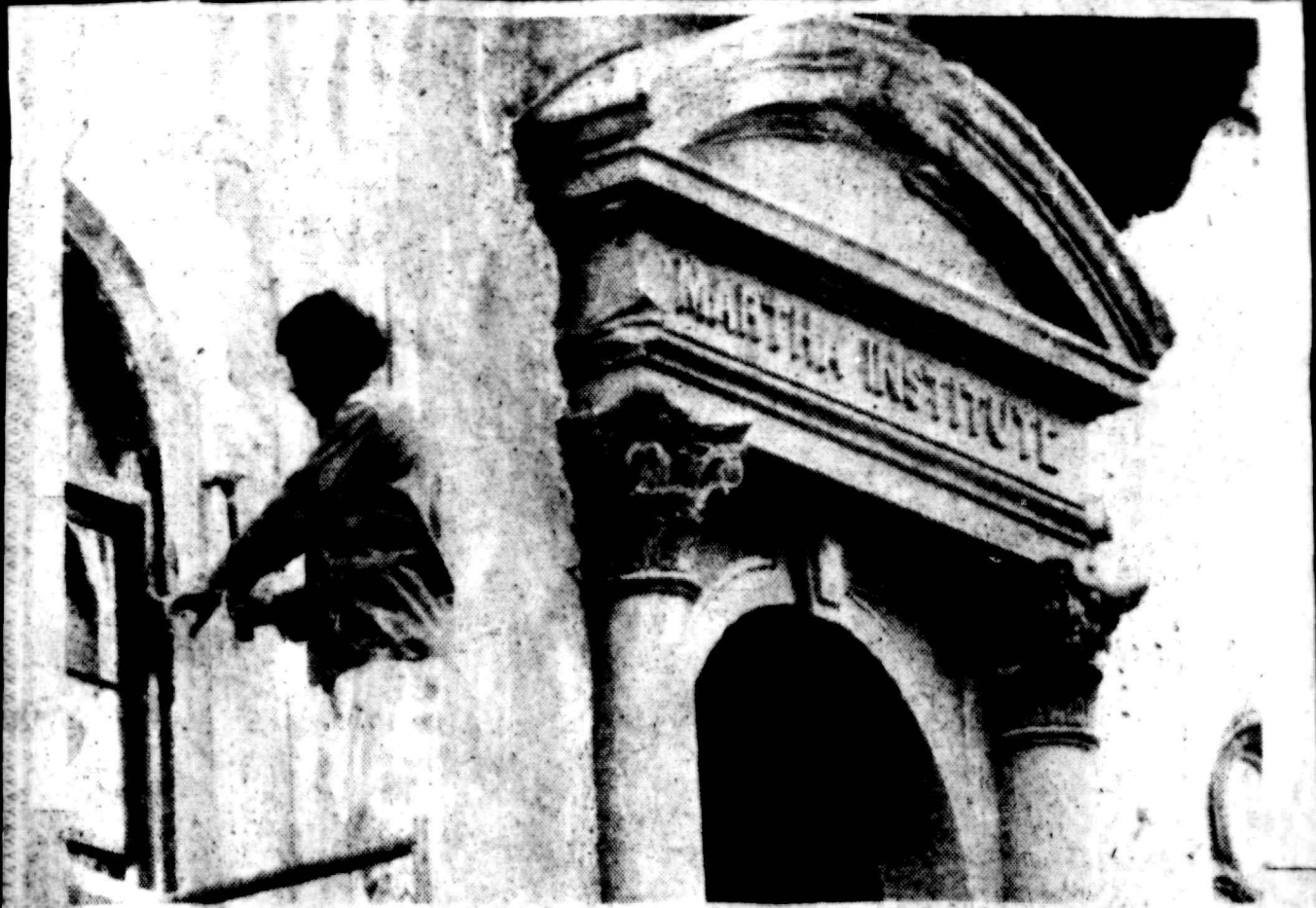
Frank Meola frames out new rectangular window, replacing rounded window built into religious edifice 111 years ago.
